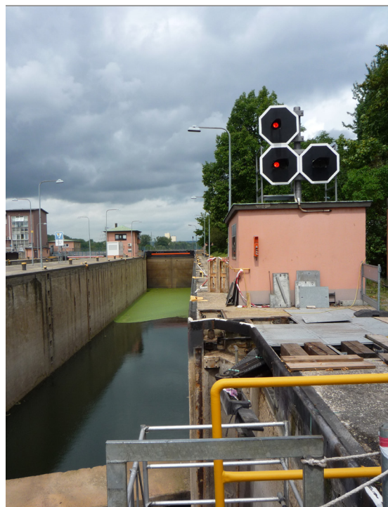
Figure 1: River lock chamber during maintenance work [Foto: Nickel/IFA]
